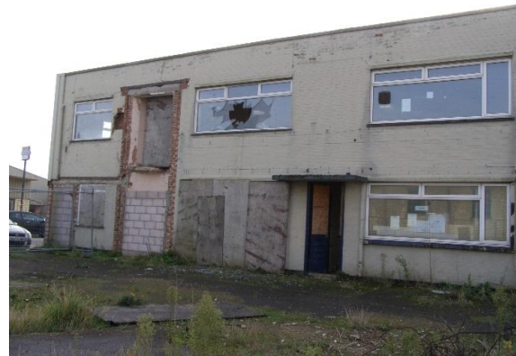
View of Office Area Prior to Works
