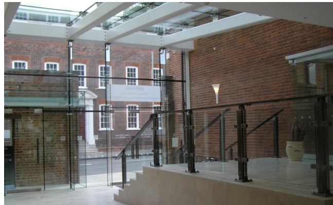
New Steel Framed & Glazed Atrium Link Structure
