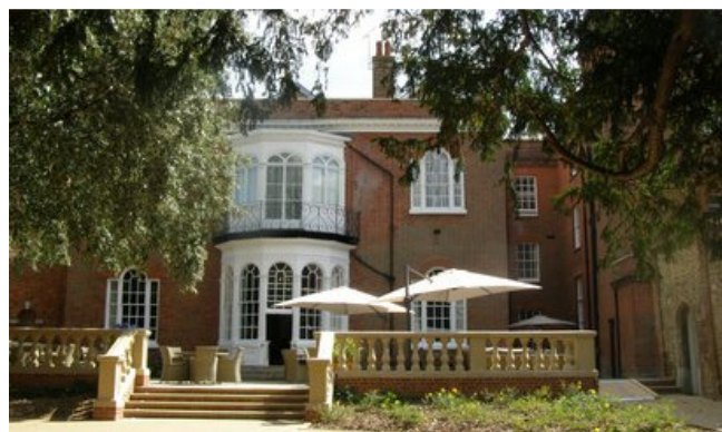
Rear Elevation & Sun Terrace
